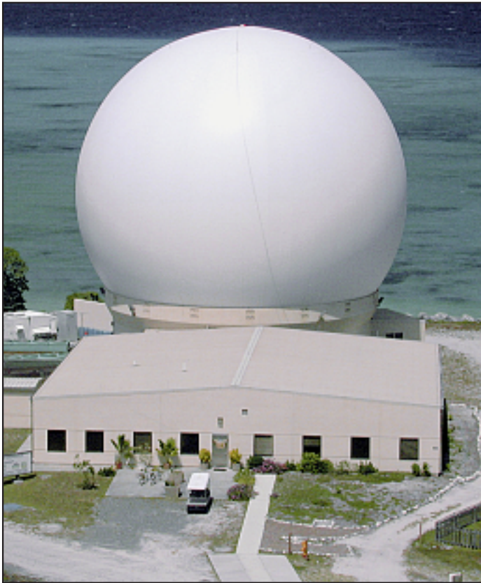
The GBR-P at Kwajalein Atoll (US Army) 0543434
